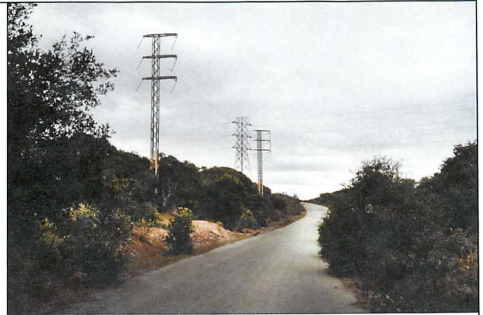
View along Gigling Road near where power lines cross.
